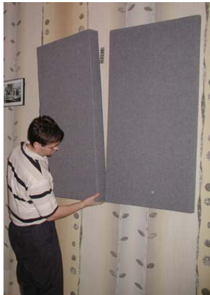
Locate absorber and diffuser suspension V-bars
